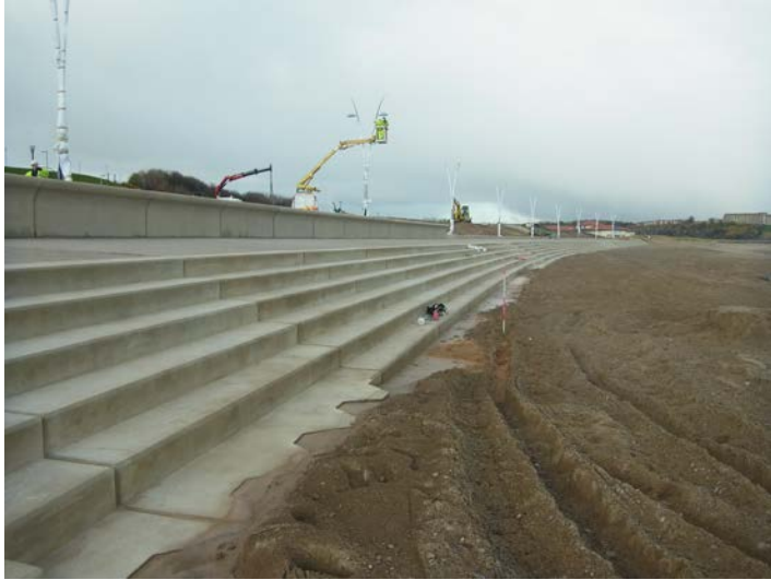
Plate 1 – Survey photograph 1bSS3_20131119_N1.JPG (Shows new and realigned Littlehaven seawall)
