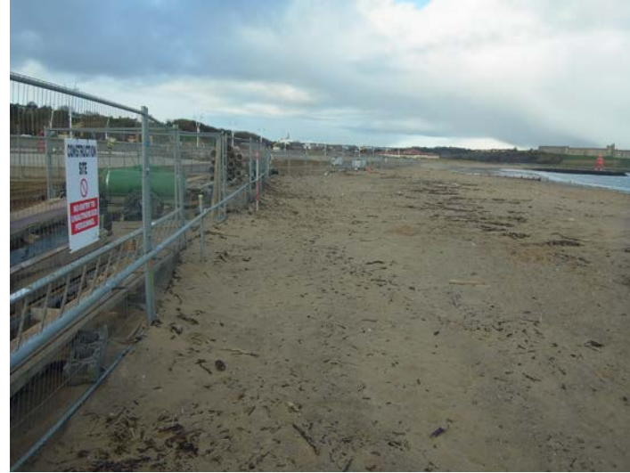
Plate 2 – Survey photograph 1bSS4_20131119_N1.JPG (Works underway to Littlehaven seawall)
